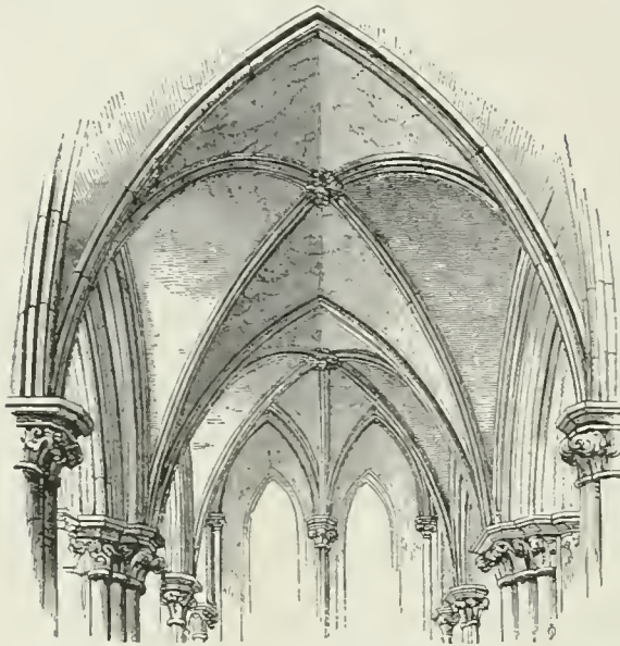
RIB. *FIG. 1: EARLY RIBBED VAULTING WITH ONLY THE ESSENTIAL RIBS, VIZ., DIAGONAL RIBS (OGIVES) MEETING AT THE CENTRAL BOSS; TRANSVERSE RIBS SEPARATING THE VAULTING SQUARES; WALL RIBS (FORMERETS) ON RIGHT AND LEFT; THE COMPARTMENT IN THE DISTANCE IS, IN PART, IN SEXPARTITE VAULTING; SALISBURY CATHEDRAL.
